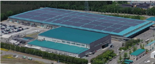
Photovoltaic (solar) power generating facilities at Sakata Plant
