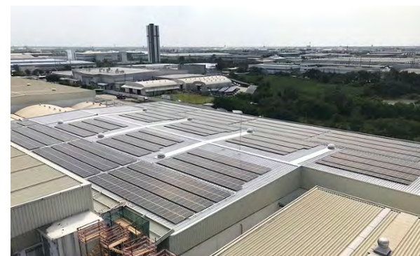
Solar power is installed at the Kao Industrial (Thailand) plant
