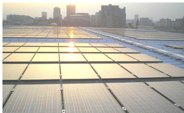
Solar photovoltaic panel installed on the roof of the Logistics Center
