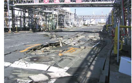
Kashima Plant suffered damage from liquefaction
