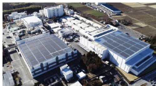
Photovoltaic (solar) power generating facilities at Tochigi Plant
