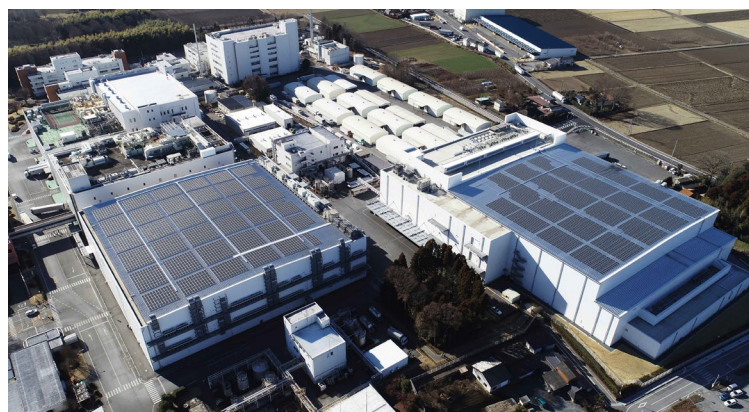
Solar panels on Kao's Tochigi plant in Japan
