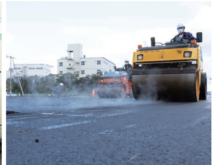
Measuring the strength of the asphalt modifier in the lab, and a paving project using the product. Adding just 1% asphalt modifier improves the durability of the asphalt pavement approximately five-fold.
