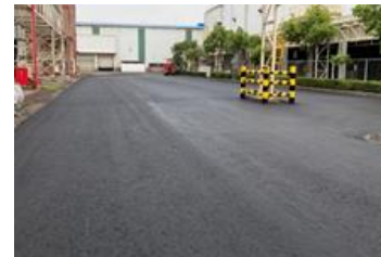
Test construction was conducted in Taiwan for overseas rollout of highly durable asphalt modifier using waste PET.
