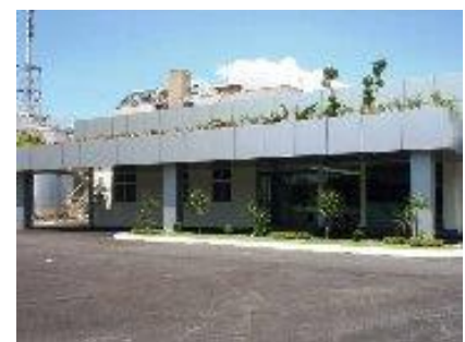
The new Fatty Chemical (Malaysia) offices
